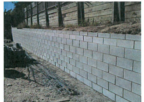
Smooth Face CMU Wall
