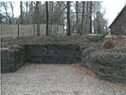
Railroad Tie/ Wood Wall
