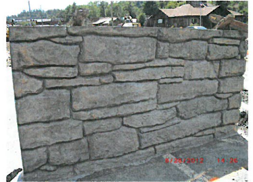
Concrete Form Liner Wall
