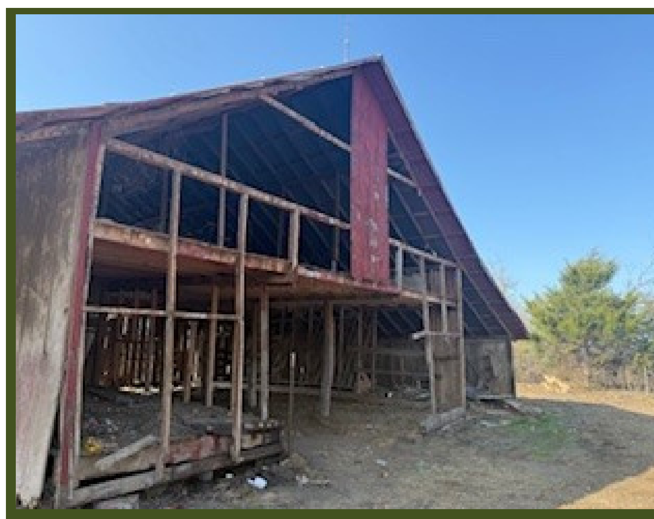
FM 1141 / ALMA WILLIAMS PARK BARN REMOVAL
